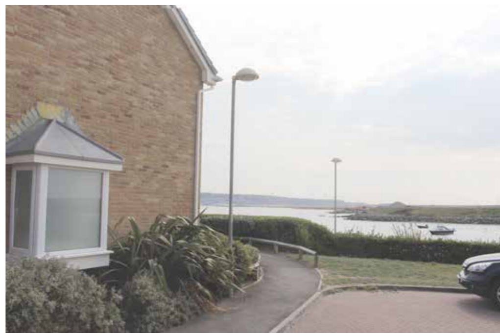
4. View of existing property (23) from neighbours' (21)
