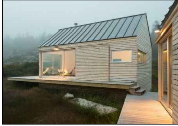
Image A Zinc Roof Cladding With Upstand Profile
