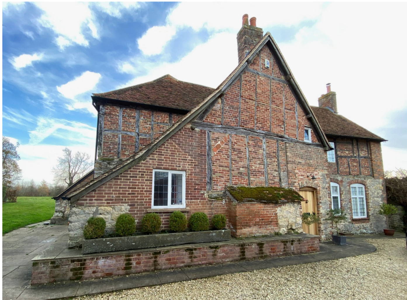
The front/north elevation of Pasture Farm House.
