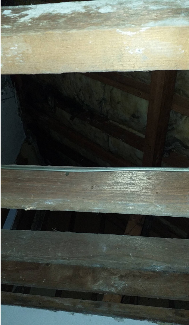
Photograph from the ground floor looking up into the roof void
