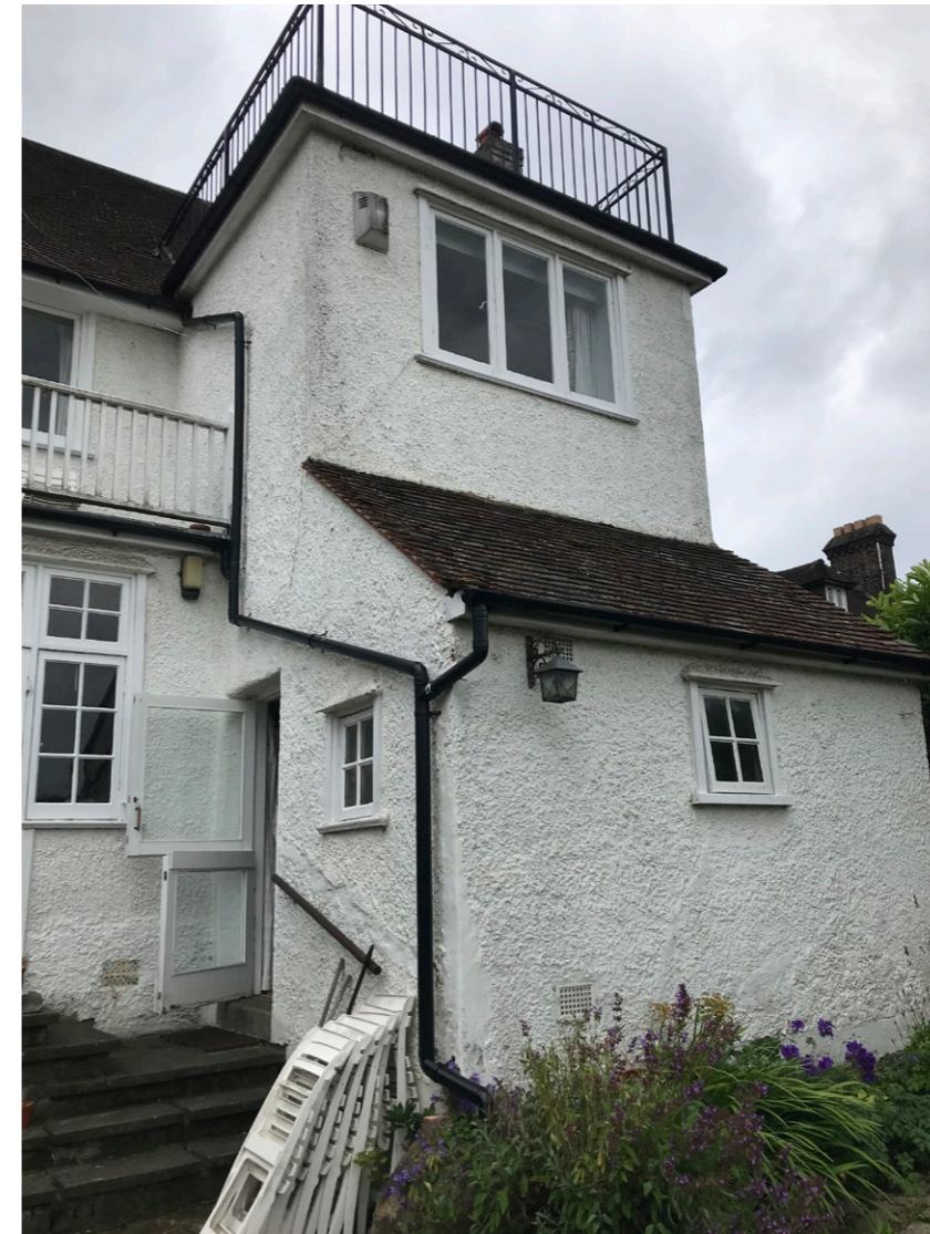
View 4 - Close-up view of existing rear pantry on ground floor
