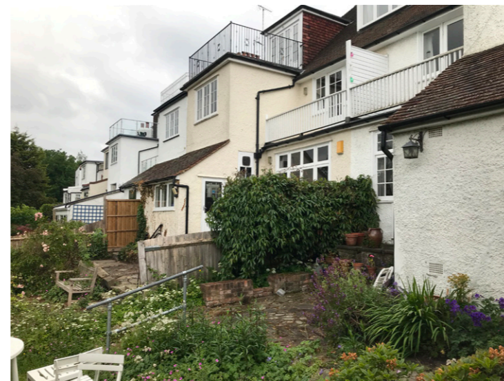
View 3 - Existing rear view towards adjoining neighbour No. 20 showing existing balconies.
