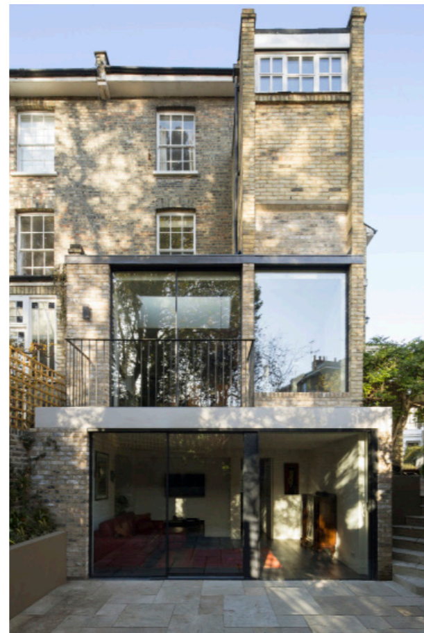
Richmond Crescent, Barnsbury, London
