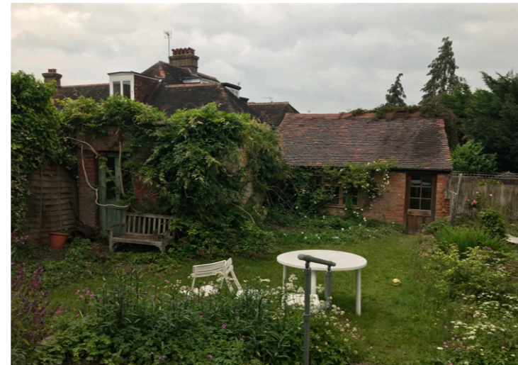
View 2 - Existing rear garage outbuildings
