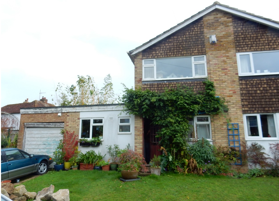
VIEW OF EXISTING PROPERTY FACING ONTO APPLETON
