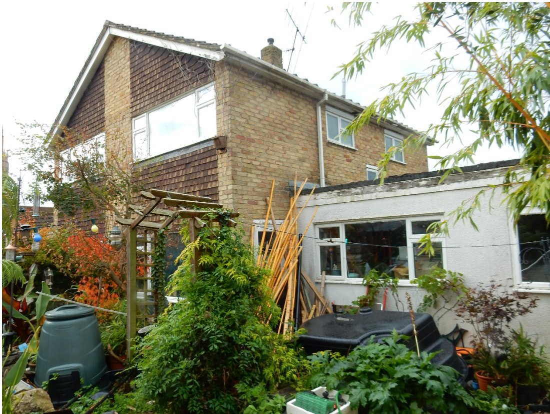
VIEW OF EXISTING REAR ELEVATION ON REAR GARDEN
