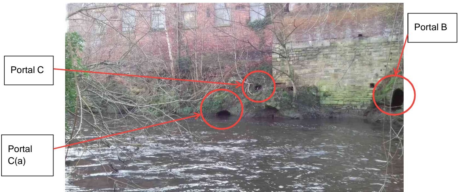
Photograph 2: Portal C and C(a) from the northern bank of the River Mersey
