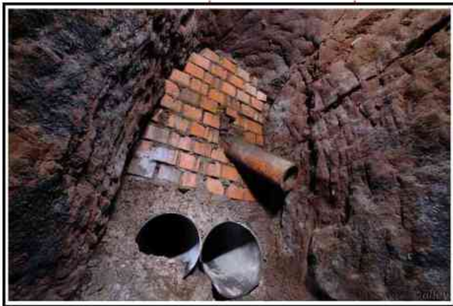
Photograph 9 – Brick headwall and pipes within Binns' Deep
