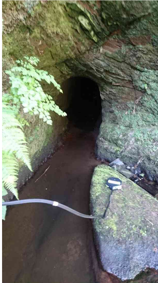
Photograph 6 - Portal F (Binns' Deep)
