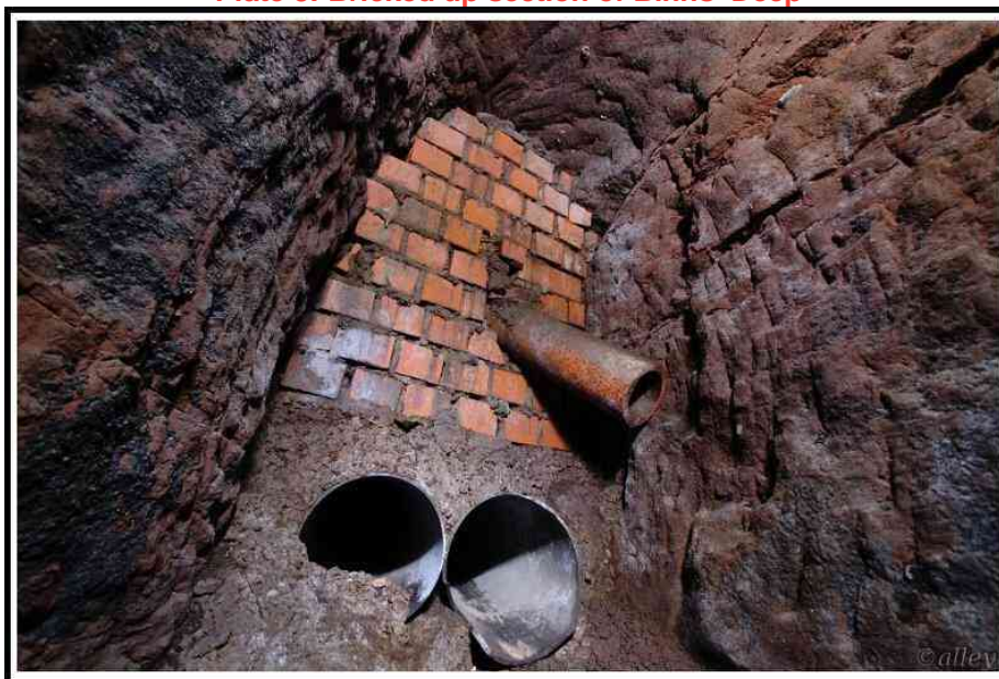
Plate 8: Bricked up section of Binns' Deep
