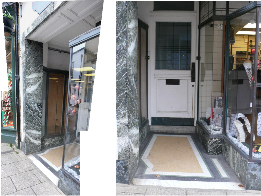
Recessed entrance to flat above, with shop display case to the left
