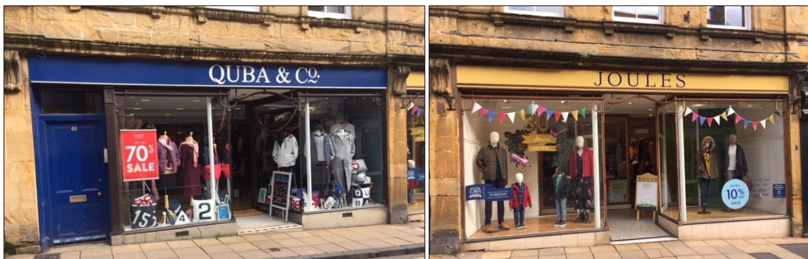
Fig.2 Nos 65 & 67 Cheap Street Quba & Co and Joules shopfronts.
