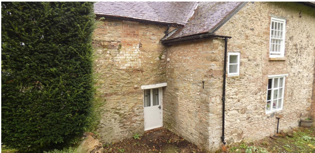
Blocked up windows and doors attest to the various modifications the Rectory has experienced over the years
