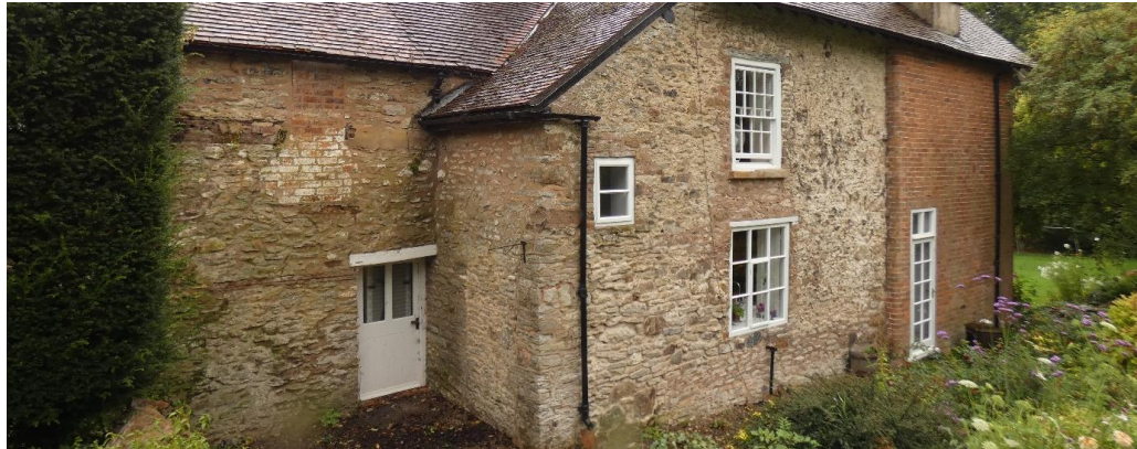
Site of proposed lean-to viewed from the north west
