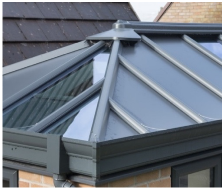
Typical Roof finish
