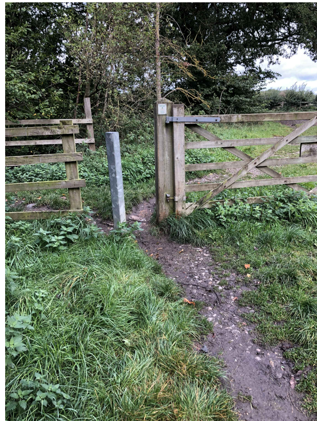
Existing Access Gate No.1
