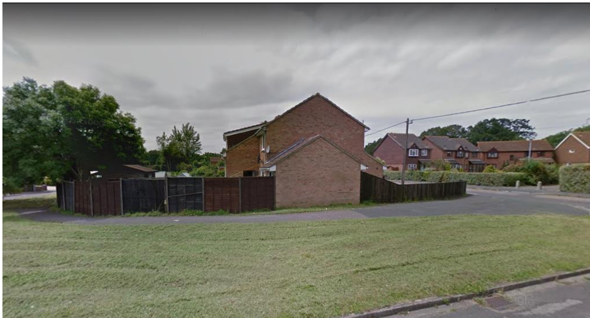
BELOW: GOOGLE STREETVIEW SIDE ELEVATION
