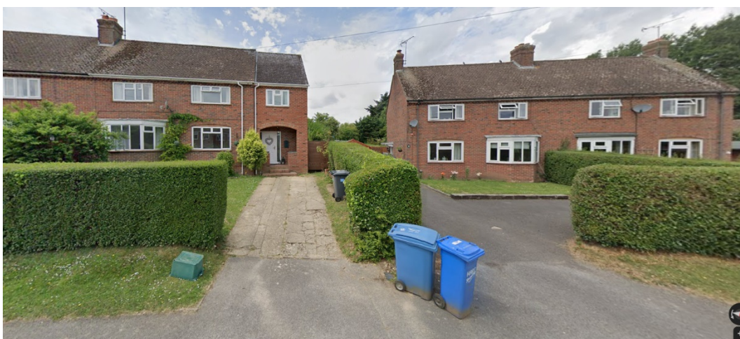
Fig 8 – Semi-detached dwellings at 17-20 Chaundlers Croft
