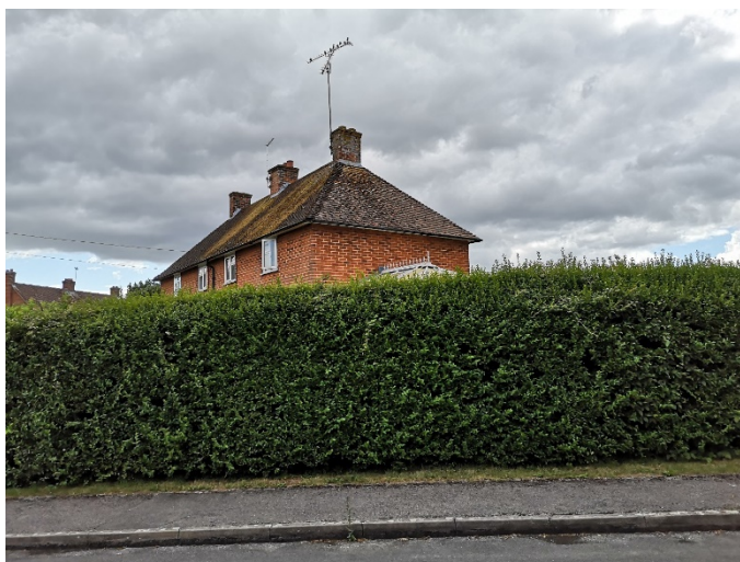
Fig 3 – View towards the side elevation of 28 St Cross Road from Chaundlers Croft
