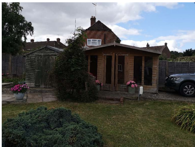
Fig 6 – View towards the outbuildings to be removed
