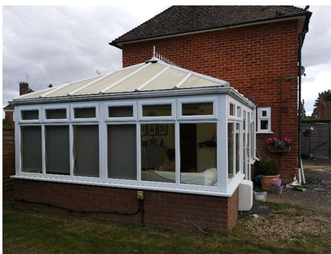
Fig 5 – View of conservatory to 28 St Cross Road to be removed
