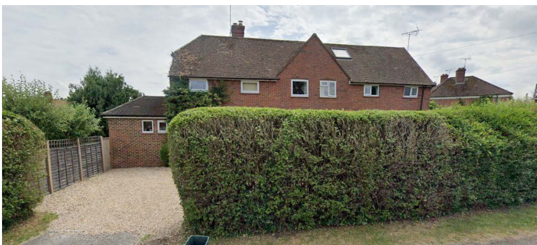
Fig 7 - Neighbouring dwellings – 14 & 13 Chaundlers Croft
