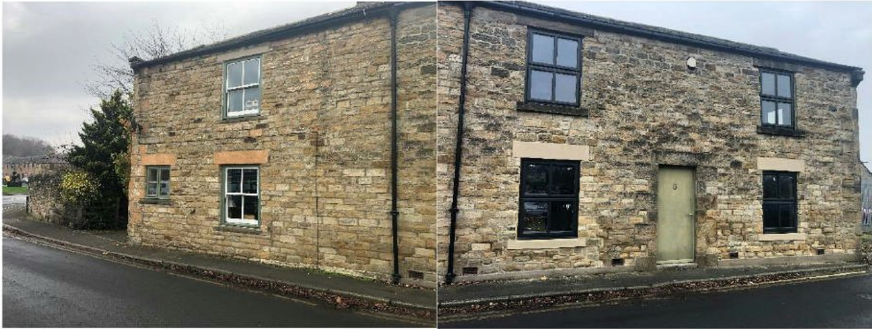
Left: Adjacent dwelling, patchwork of green and white painted timber windows Right: Application site, dark grey uPVC
