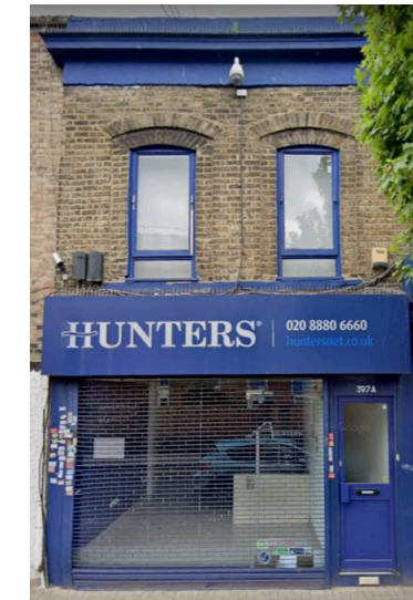
Front Elevation Photo as Existing - NTS
