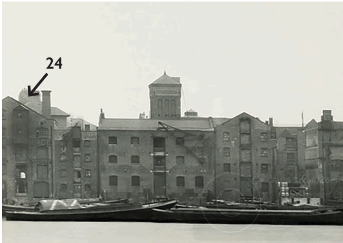
NORTH BANK OF THE RIVER THAMES - 24 NARROW ST FAR-LEFT
