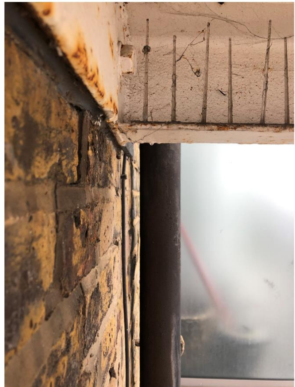
Figure 13 - Close up of the brickwork moving forwards
