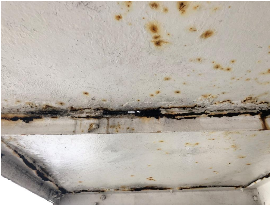
Figure 5 - Underside of fifth floor deck
