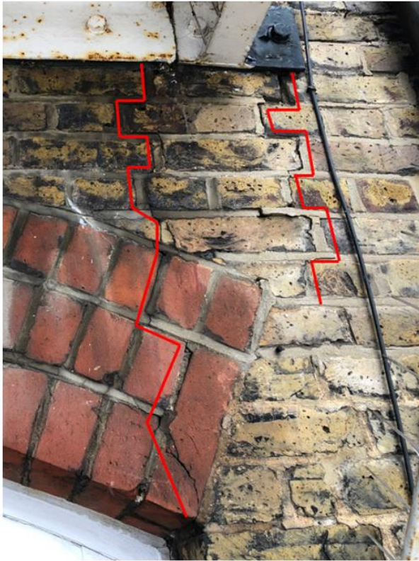
Figure 12 – Displaced brickwork at structural frame level (balcony 4 th floor)
