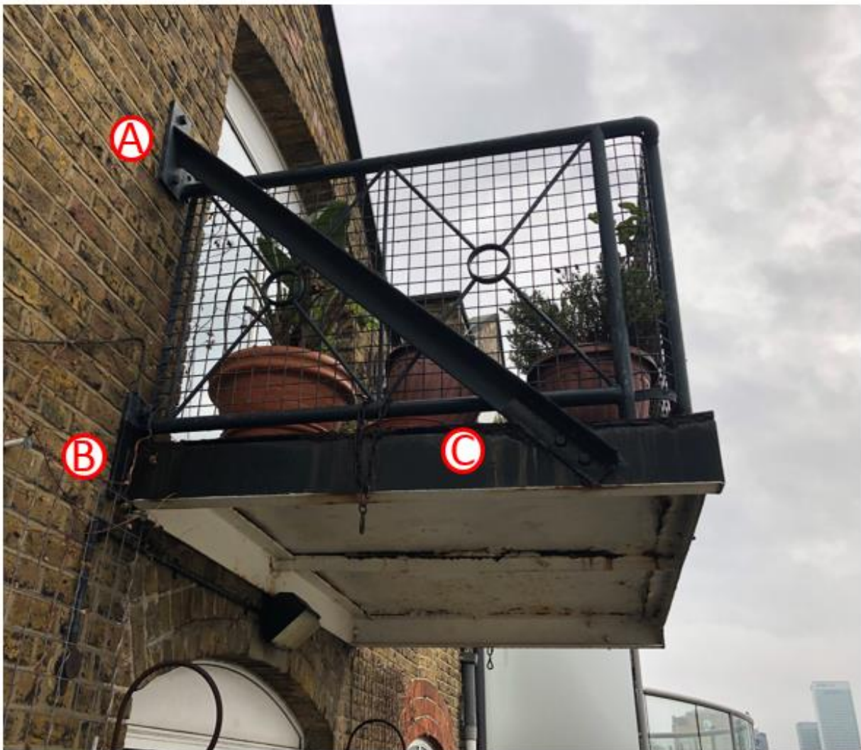
Figure 1 - Fifth floor balcony
