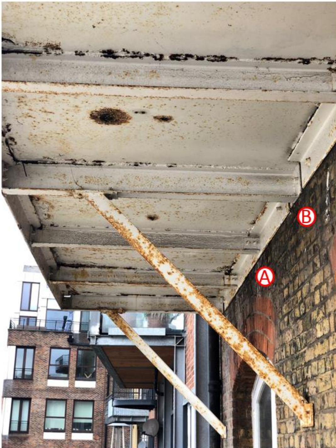
Figure 9 - Underside of fourth floor balcony deck, with diagonal propping
