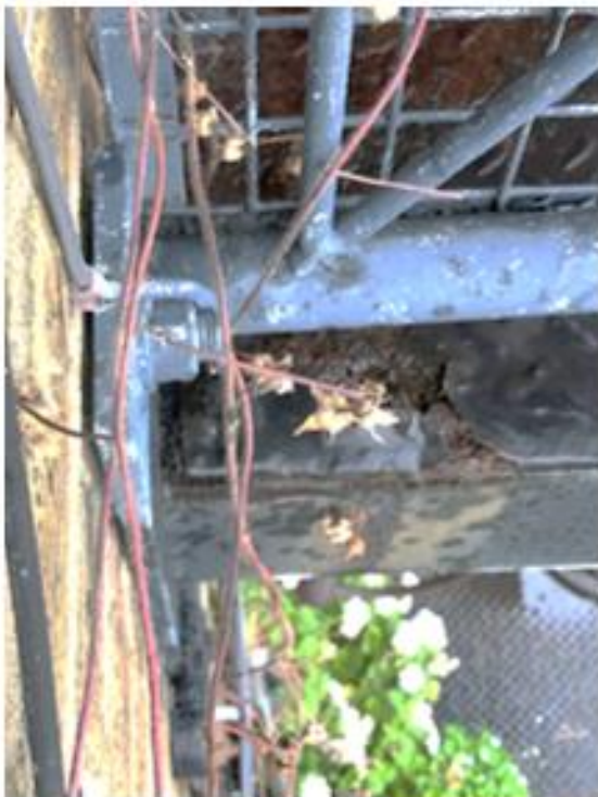
Figure 4 - Corrosion on fifth floor deck, (Top Left) across surface, (Top Right & Lower Right) Butted region of plates in centre of balcony, (Lower Left) design encouraging water to drip and collected at edge of plate.
