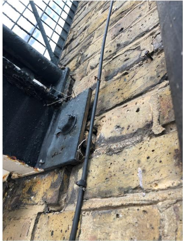
Figure 12 – Displaced brickwork at structural frame level (balcony 4 th floor)
