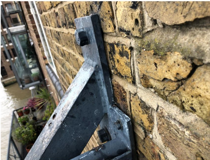
Figure 3 - Diagonal bracing to brickwork fixing (left) and Cantilever brickwork connection
