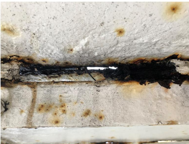
Figure 6 - Central support (Left) and the material flaking away (right)
