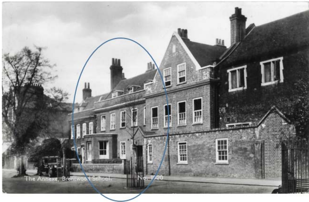
Figure 8. Photograph of the School House shortly after 1926. In the foreground, the extension was rebuilt as a 3-storey block with a gabled frontage linking School House with the Old School building. This extension provided new dormitories and changing rooms and the photograph is entitled 'The Annex' indicating it may have just been completed." 2
