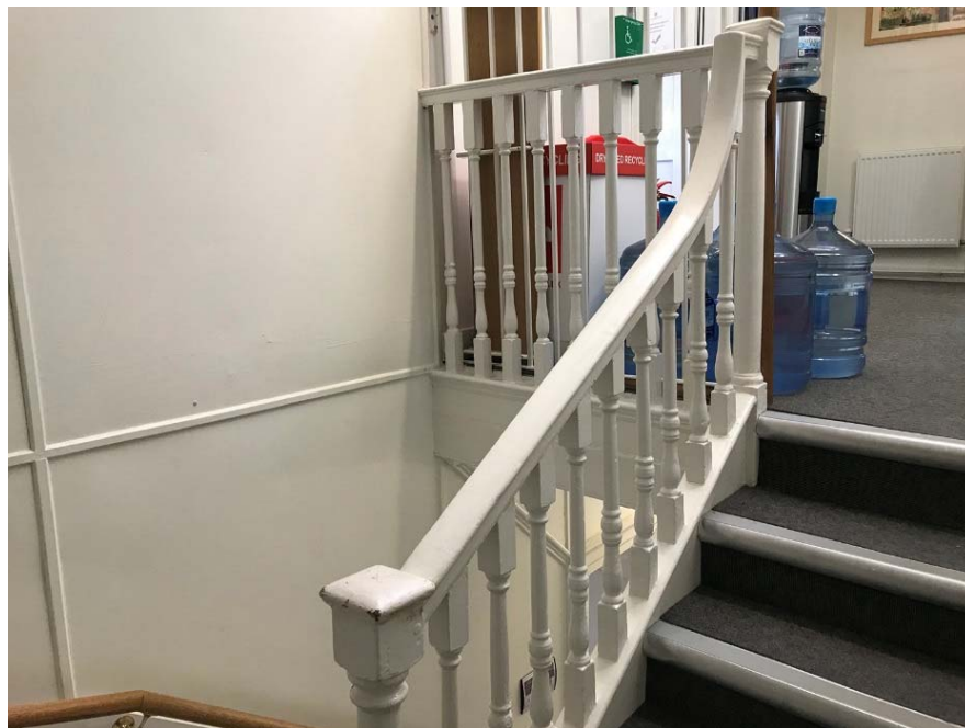
Figure 11. Original C18 staircase is retained and walls lined for fire resistance.
