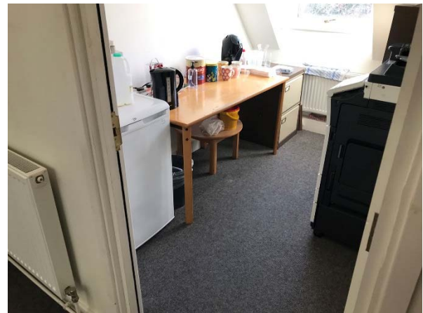
Figure 14 (above right). Looking from the Landing into the Store/Kitchenette. This was converted from a Bathroom in 2013 and it is proposed to reinstate a water supply into this area.
