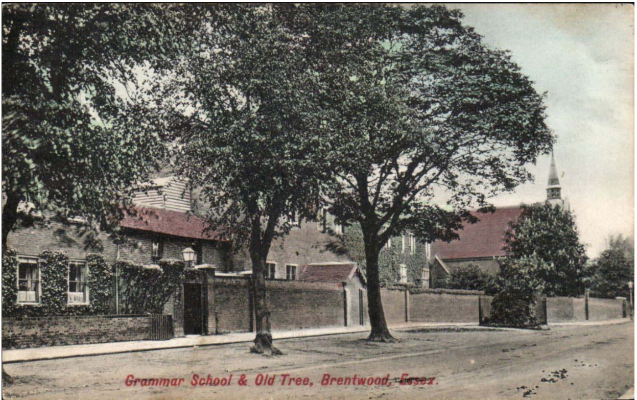
Figure 6. School House (left) looking from the north, showing its fenestration and extension of Mid-C19. The photograph is circa 1905.
