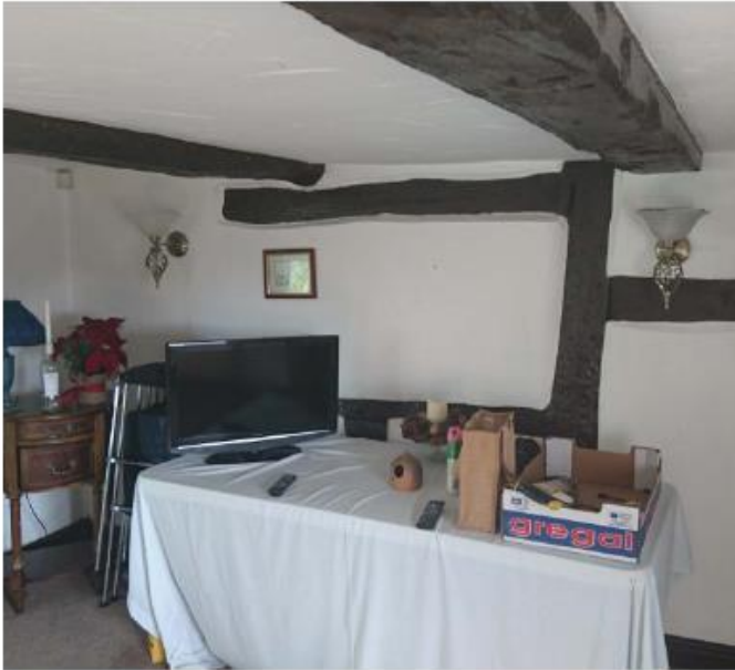
Evidence of original oak beam in rear sitting room which has been severed over time
