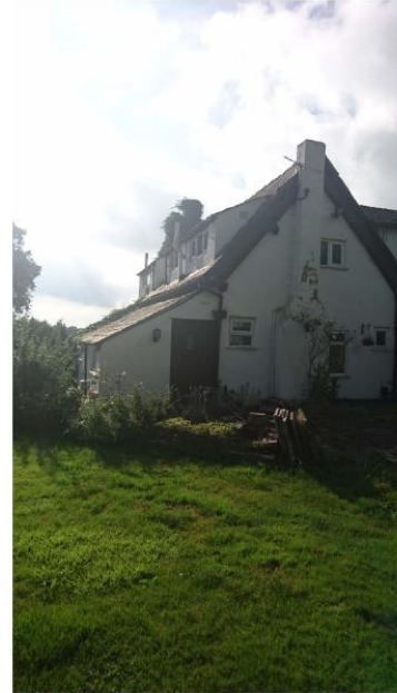
External image of A frame
