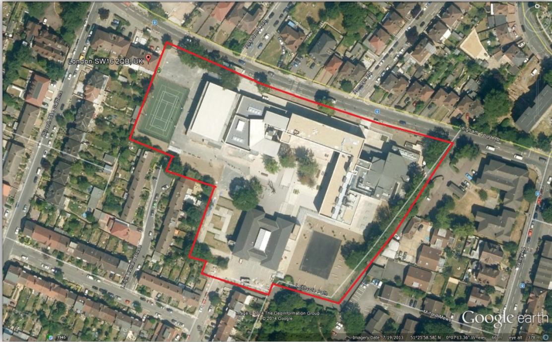
Aerial photograph of the site: Google Earth Imagery
