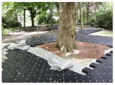
Substituting traditional compacted stone infill with ArborRaft or Cellweb a suspended pavement foundation sub-bases, will reduce the need for excavation and limit the weight of material build up and enable the formation of porous hard surfacing, which limits compaction of root zone within RPA.
