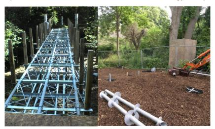
**Example 2 – Thrust or Bored Piles**. Small plant piles can be installed within Root protection area. To enable heavy buildings to be supported several smaller piles can be connected to form a pile cap providing improved support as shown below.
