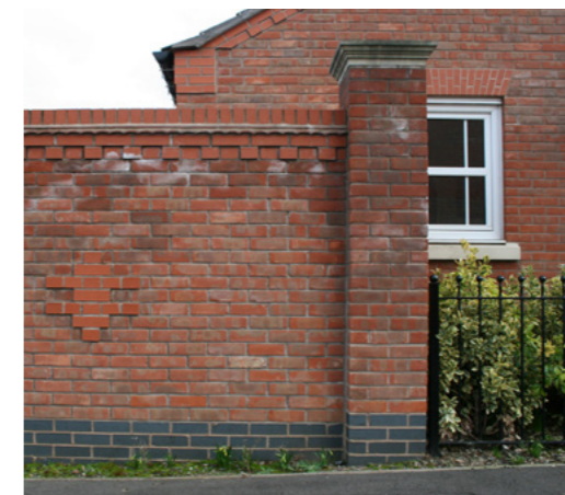
Brick Wall with Piers
