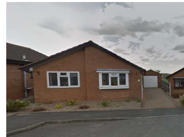
Single storey style property on Top Pingle Close
