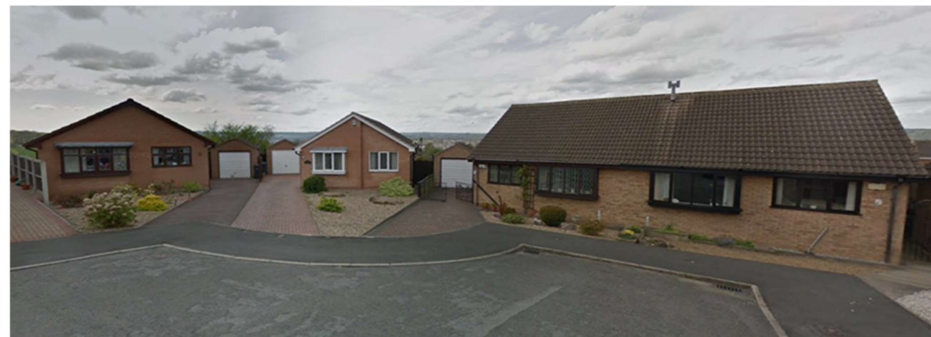
Single storey properties along Top Pingle Close located to the north of the development site
