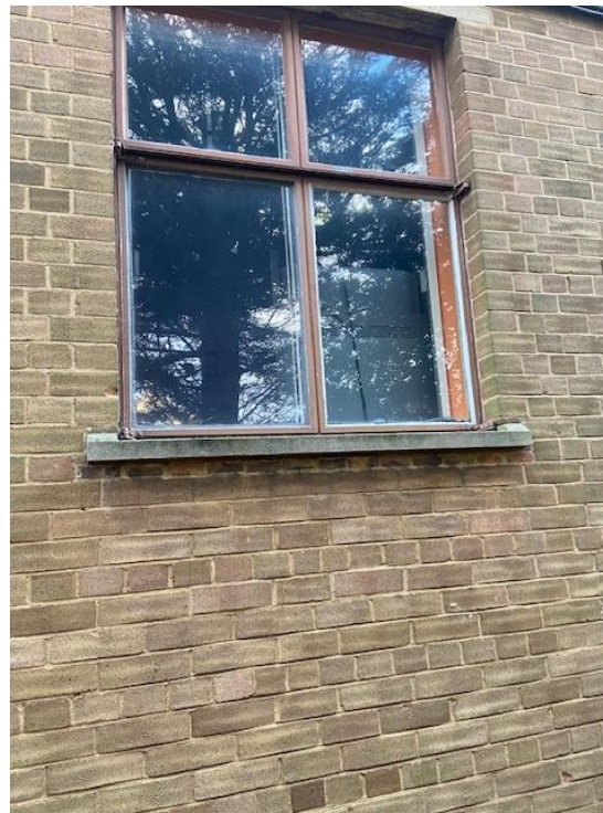
Example window being replace
