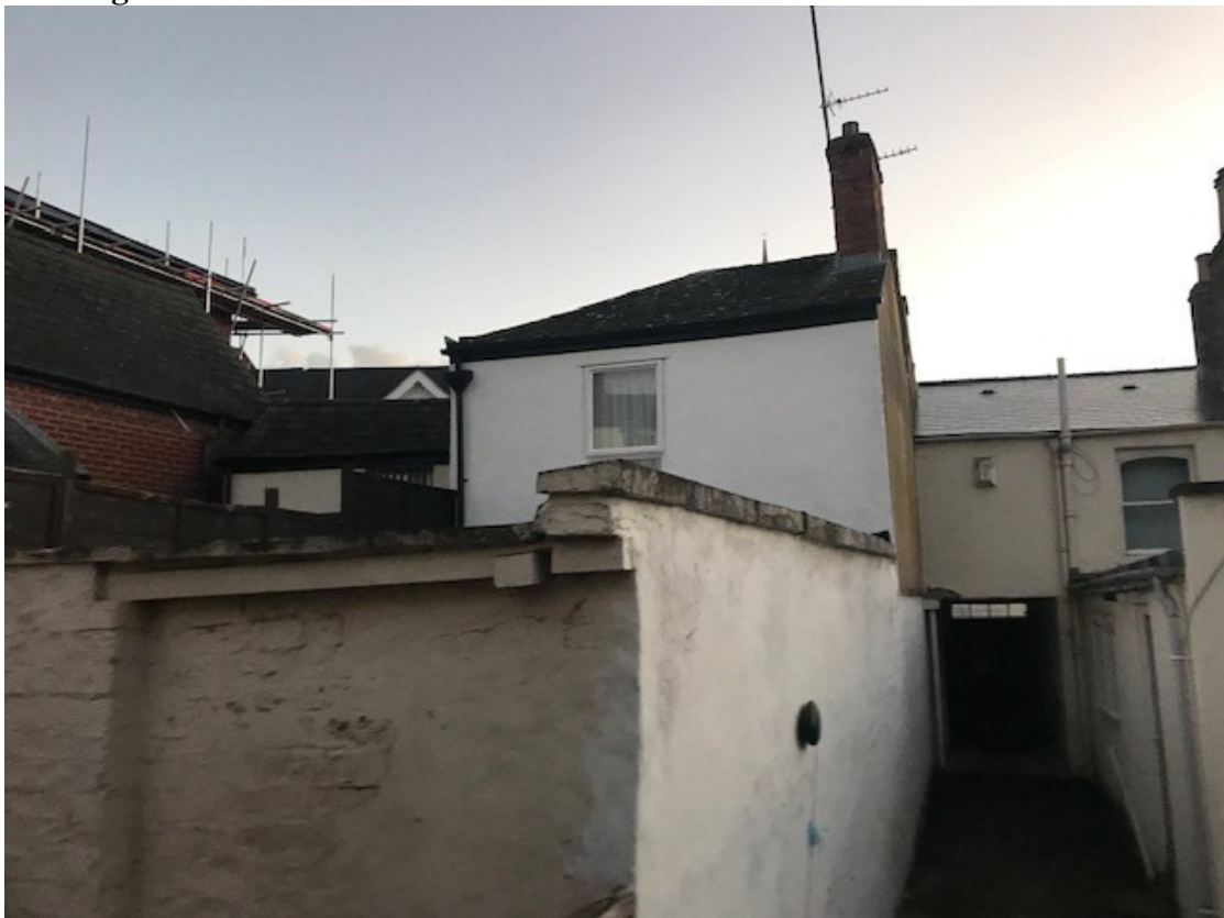
Boundary wall and rear of 17 New Street
