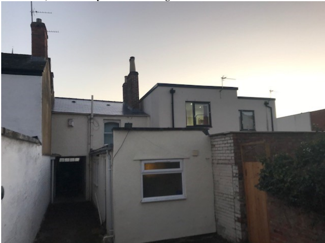
Rear of 19 New Street including side access
