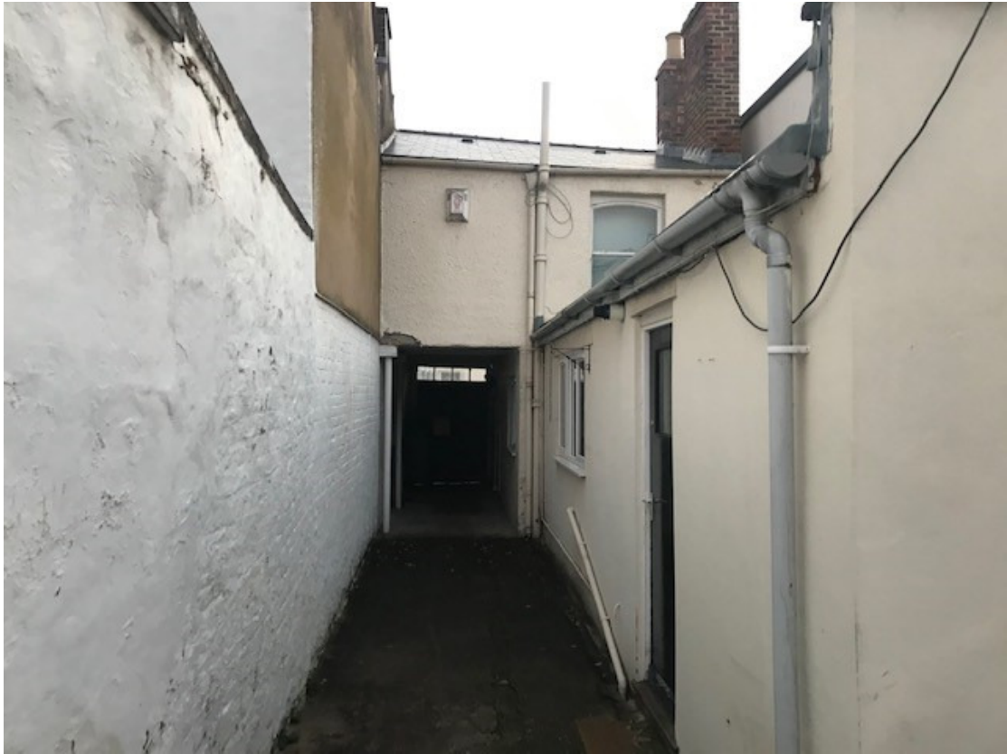
Existing access to side and rear of 19 New Street
