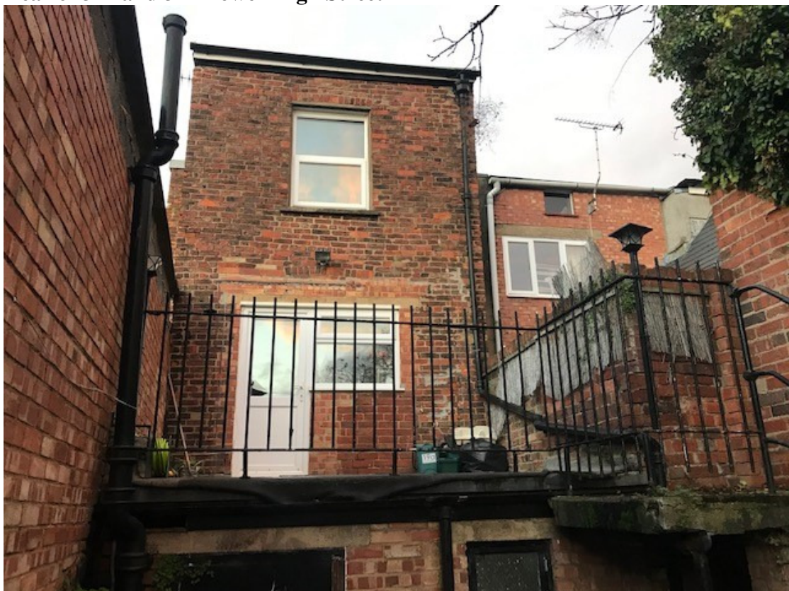
Rear of 316 & 318 Lower High Street
