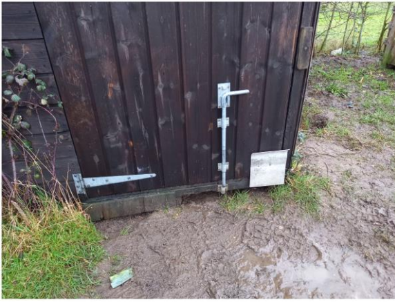
Photos of shed at Hawthorns
