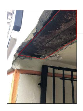
– Outline indicates existing corroded steel to be replaced.
