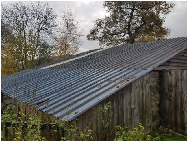
Sloping roof at north elevation.
