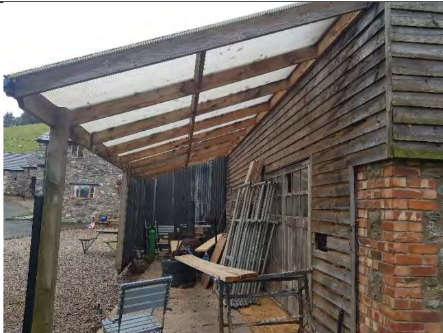
Lean-to porch at south elevation.
