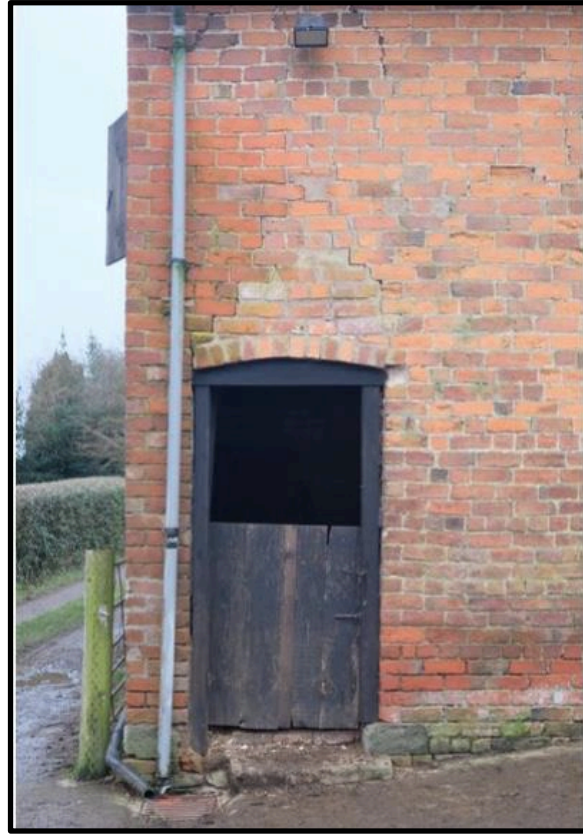
Figure 34 Southern Elevation - Barn 1 Stable Doors
