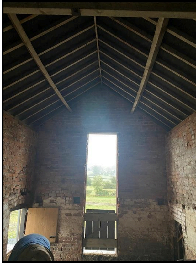
Figure 36 Barn 1 - Internal Roof Structure
