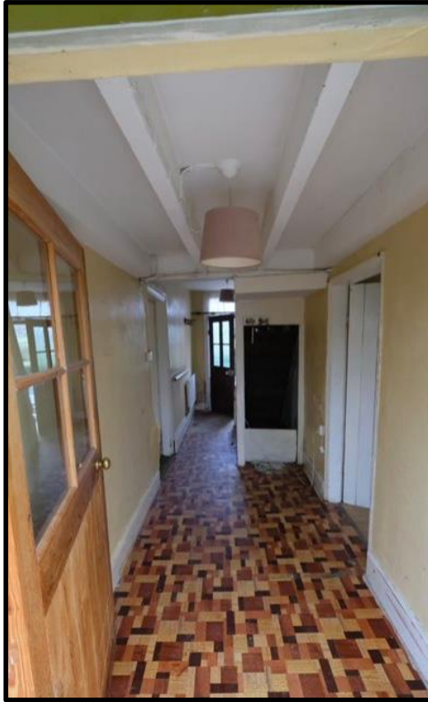
Figure 16 Internal Ground Floor Hallway
