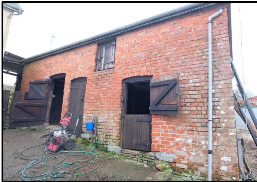
Figure 35 Southern Elevation - Barn 2 Stable Doors
