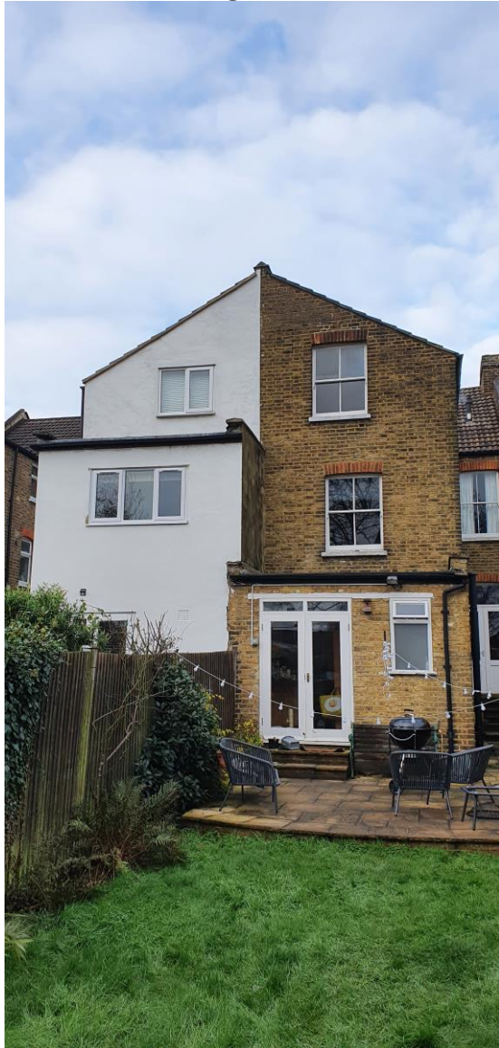
storey extension to No. 117
