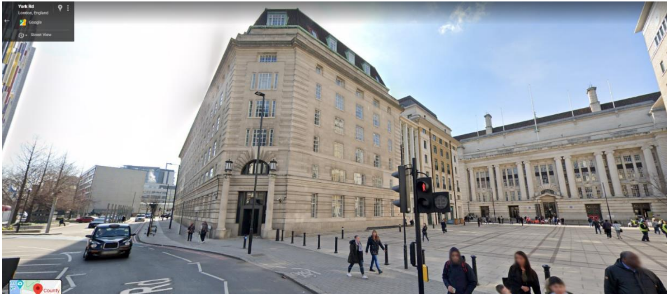
Figure 2: Street view of South Block at County Hall Apartments (Google Maps, 2020)
