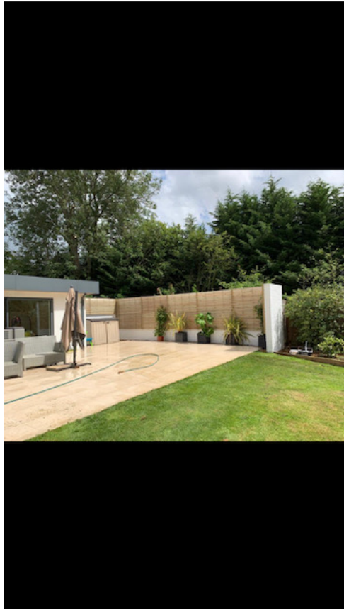
Picture of the noise attenuation wall at Liberty House
