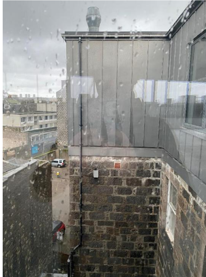
Fig36: Existing part west elevation showing existing zinc standing seam cladding and alu-clad windows
