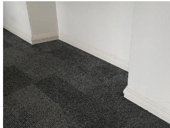
Fig15: Existing raised flooring showing what appears to be original skirting.
