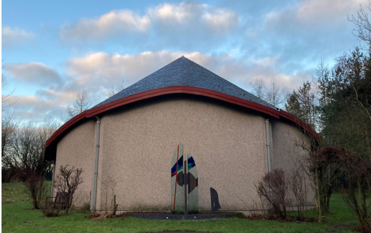
Rear Elevation (South East)
