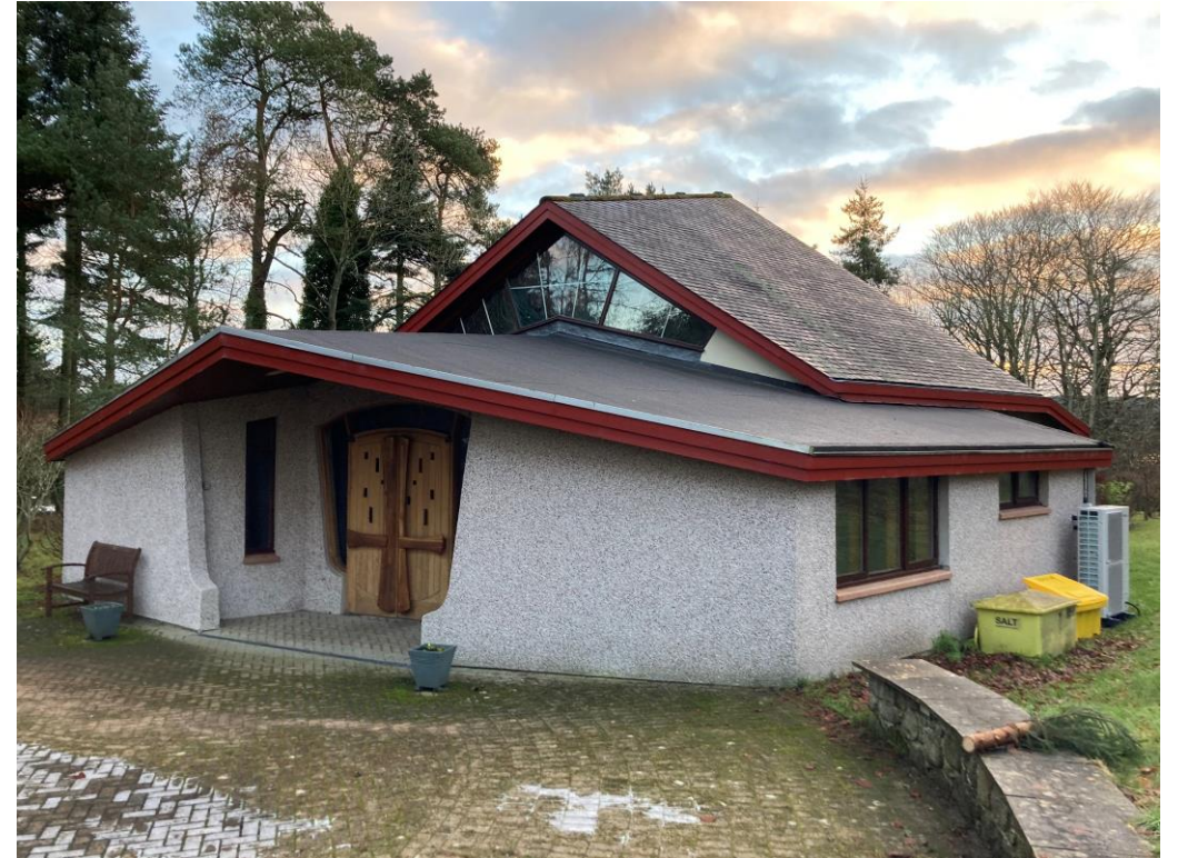
West facing view
