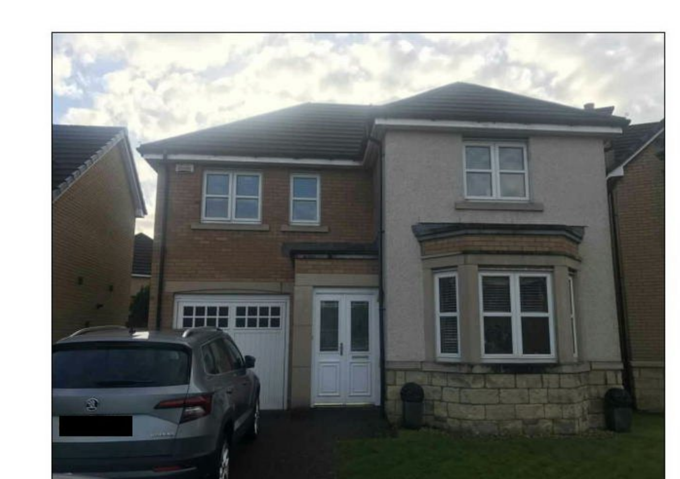
10 North Elevation (Photo) Scale NTS
