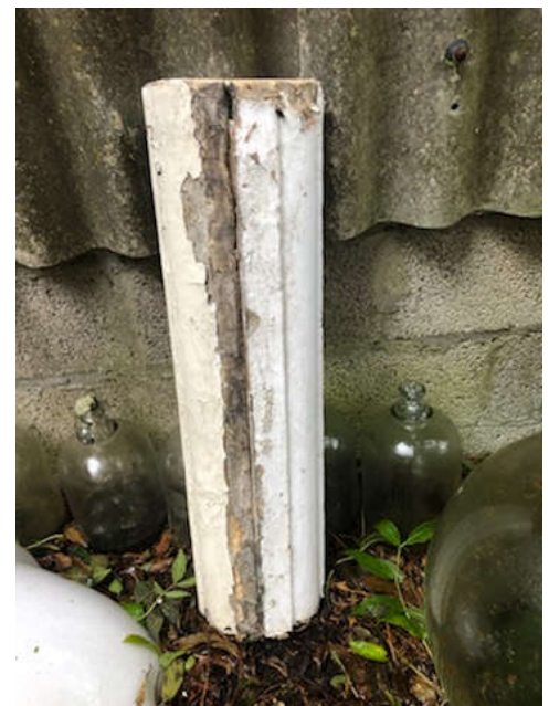
Photo 3 showing the stone mullion that has been removed but will be replaced
