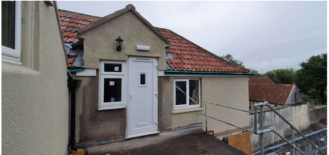
Photograph 1 showing the new dormer and escape door from the second floor hall Note that the PVC window and door will be replaced with a painted timber door and window.
