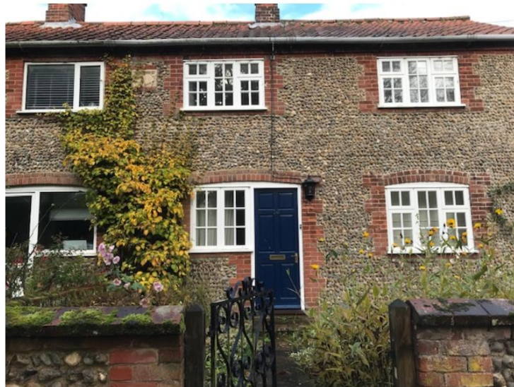
PHOTOS of 14 School Road, Saxlingham
