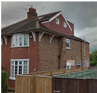
1 Westgate, Linthorpe Hip to gable with rear dormer.
