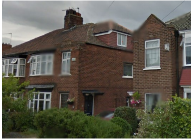
Property on Reeth road with cottage style dormer on the hipped roof
