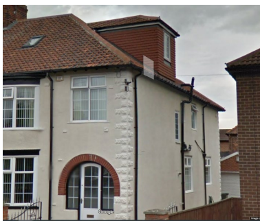
Property on Reeth road with cottage style dormer on the hipped roof
