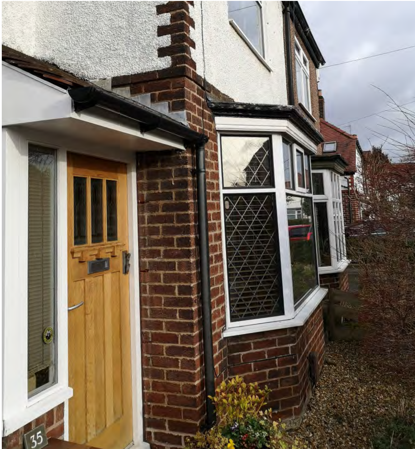
Fig. 4.3 35 Dalstone Drive - Front of Front Porch.
