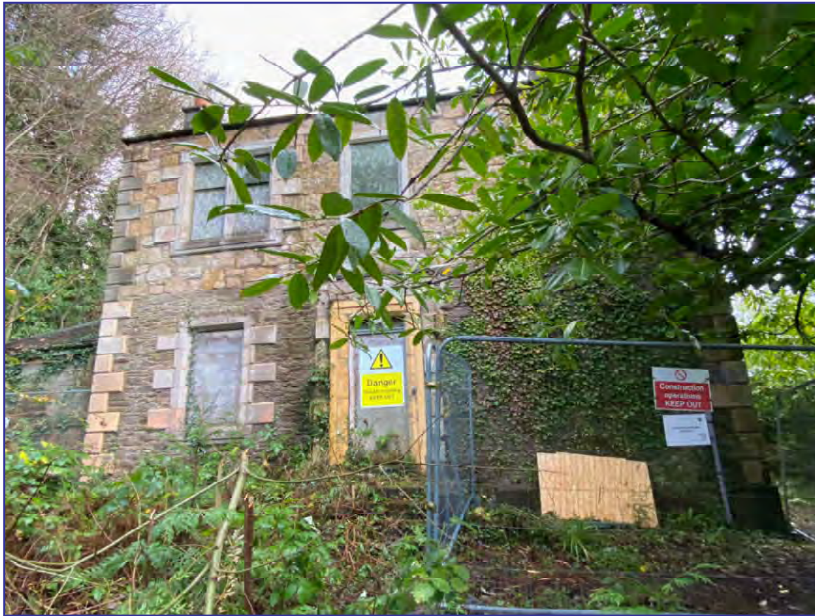
Plate 1: ESE facing view of No.105 Henderson Street (Site 90)
