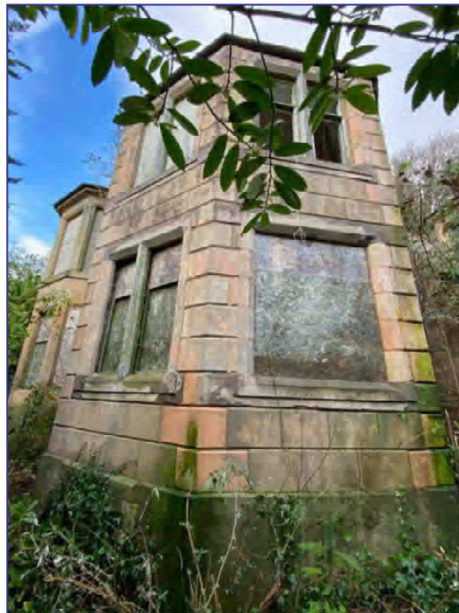
Plate 2: NNW facing view of No.105 Henderson Street (Site 90)
