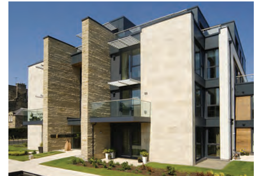
03. South Oswald Road, Edinburgh- Private Apartments (Grange Conservation Area)
