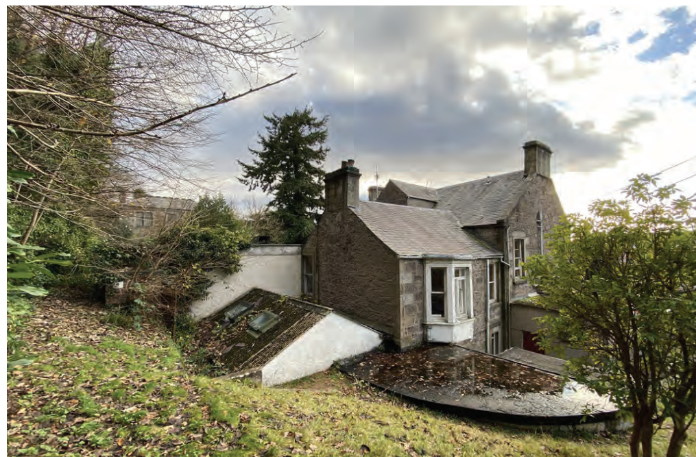
Rear of 103 (North Boundary)
