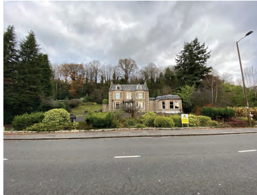
01. View From North Looking at Sites existing South Elevation
