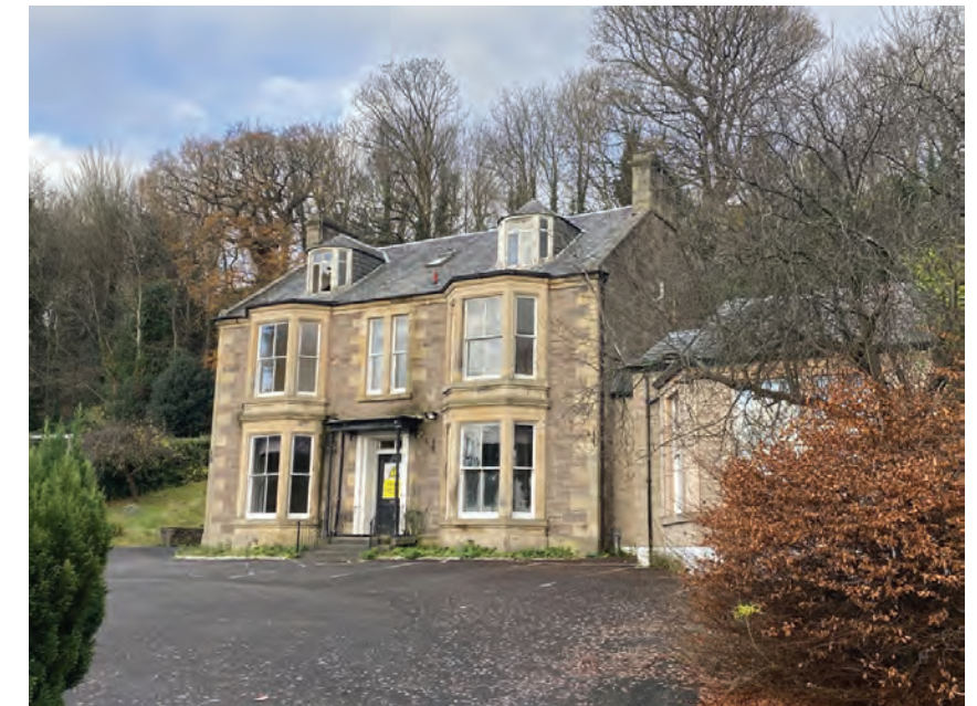
04. View From Site Looking North/West
