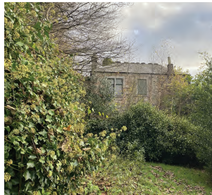
08. View Looking North East from boundary
