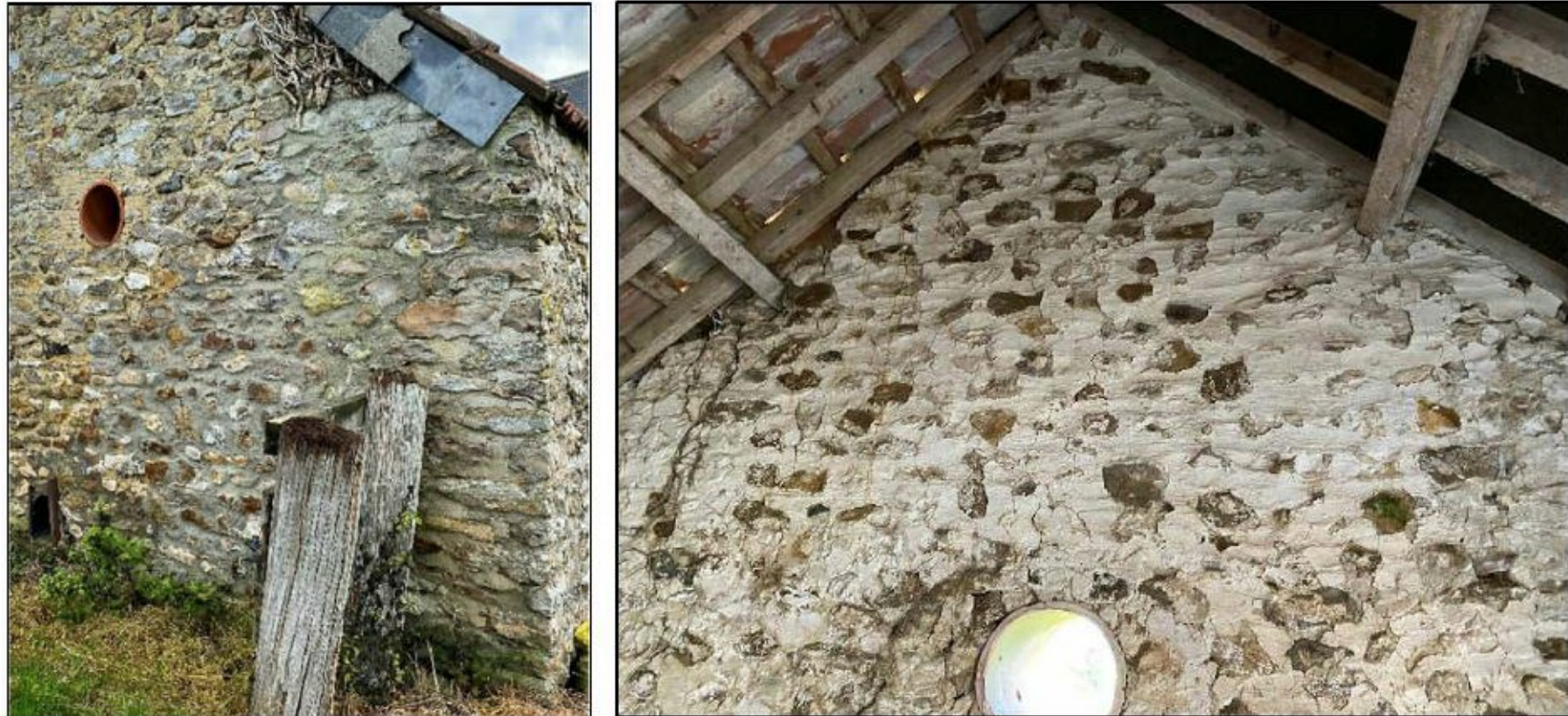
Image 6 – Evidence of previous repointing.
