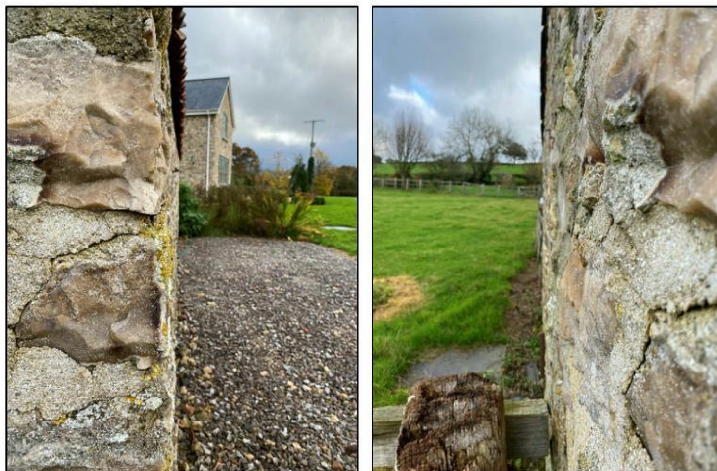
Image 5 – Exterior walls appeared straight and true.
