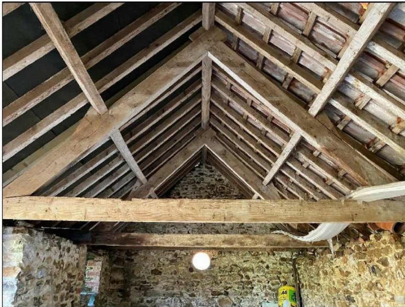
Image 2 – Timber principal roof trusses.
