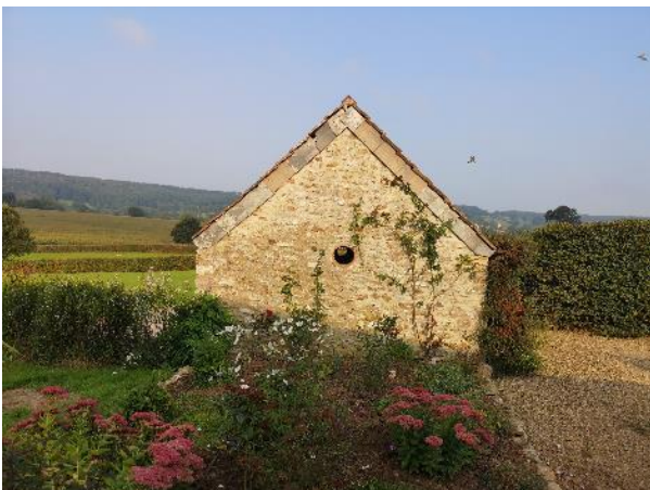
Figure 4. The south-eastern gable end of the outbuilding highlighting the hanging slate barge board
