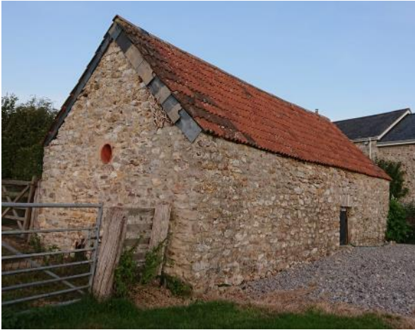
Figure 2. The south-western and north-western elevations of the outbuilding
