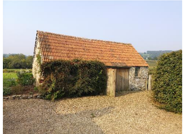
Figure 3. The north-eastern and south-eastern elevations of the outbuilding
