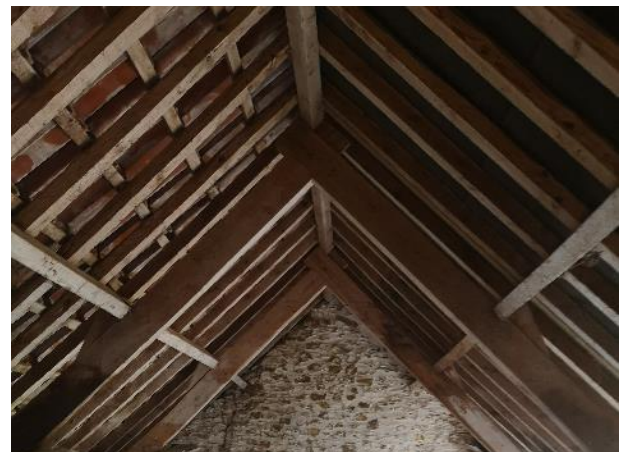
Figure 5. The internal view of the roof covering
