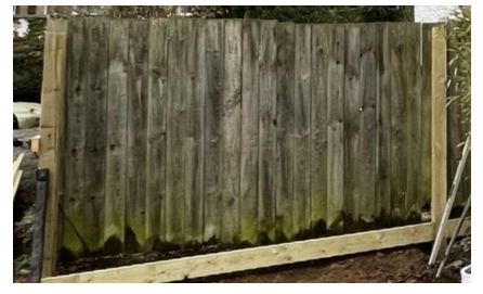
Existing close-boarded timber fence to be replicated
