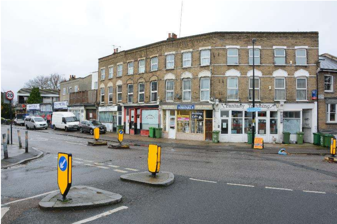
Figure 20: 1: 2-16 Evelina Road, as viewed from Gellatly Road. Facing NE.
