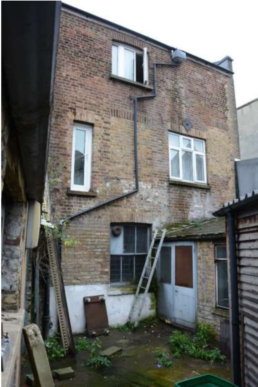
Figure 26: 7: Rear of No.10, looking towards the main building. Facing S.
